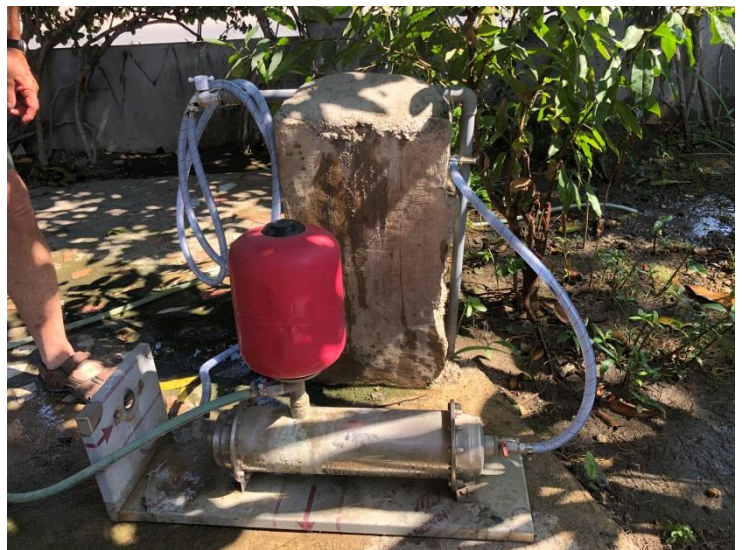
Howards filter on trial on a bore.
